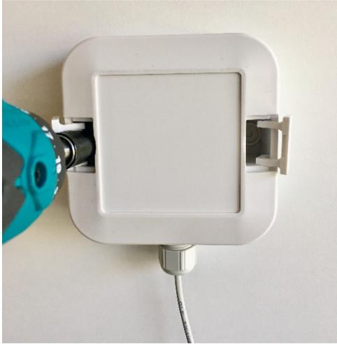
Open the hatches on the front of the casing and drill two screws into the wall.
